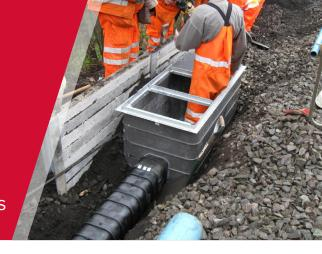
In addition, the tried and tested design of the STAKKAbox™ means that when installed, the unit will provide years of service for Network Rail. The STAKKAbox™ is not affected by diesel, ground acids, alkalines or frost – all known killers of concrete. As a structural unit it will support loadings imparted from vehicles and passing trains.
