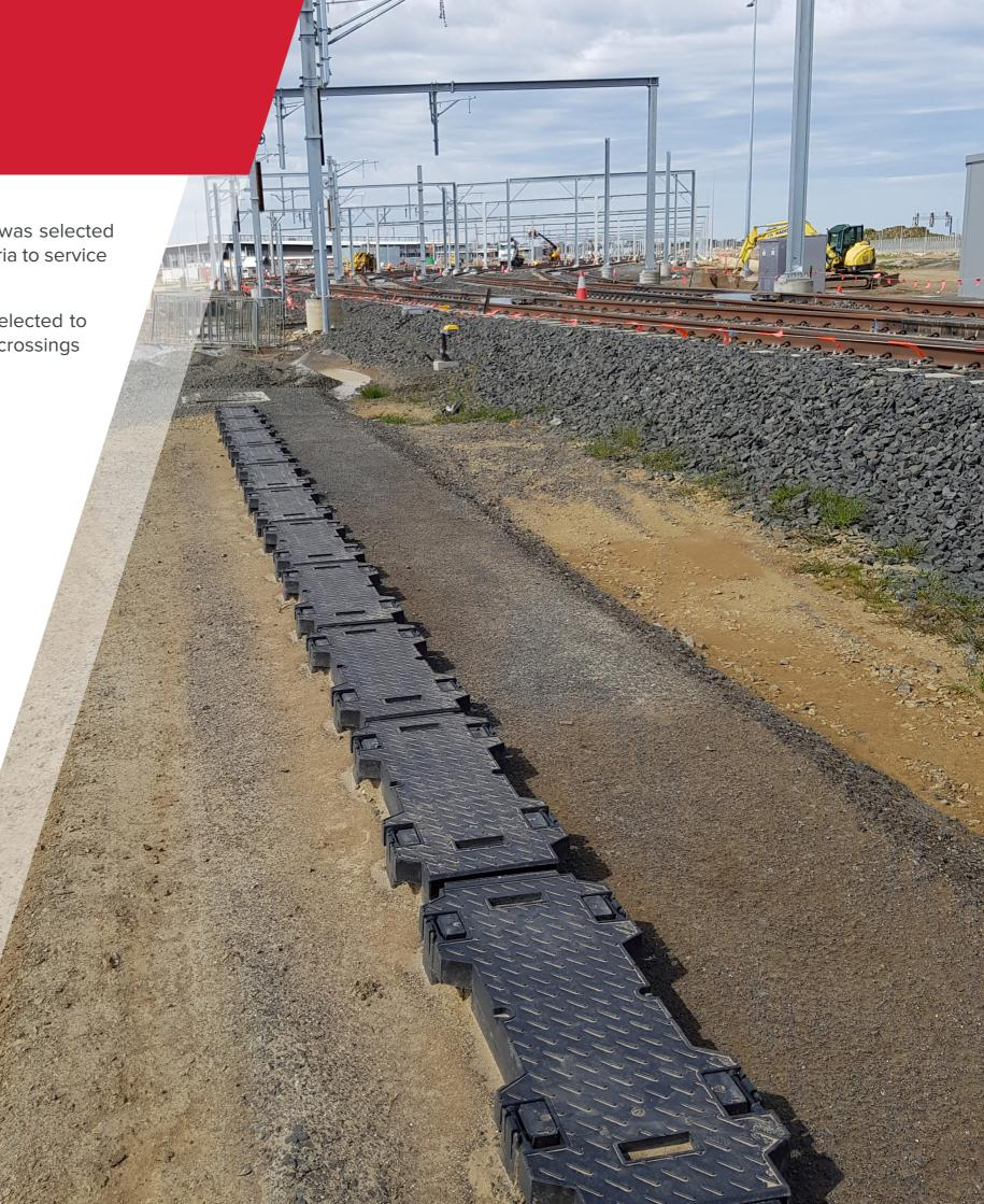
The lightweight, sturdy and secure design of the RAILduct™ provided exclusive cabling protection for the Pakenham Rail Stabling Yards project, reinforcing RAILduct™'s versatile application in rail, power and highway projects. Additionally, the timely delivery of eight (8) larger bespoke concrete chambers to the Pakenham Rail Stabling Yards project highlighted Cubis' ability to create customised product despite the tight timeframes for delivery and project completion. Together,
