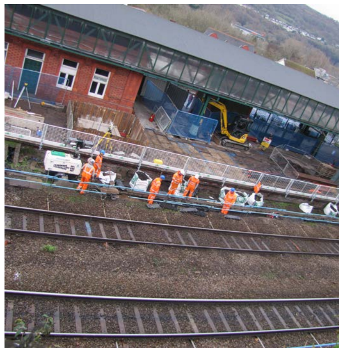
Cable Troughing - Rail
