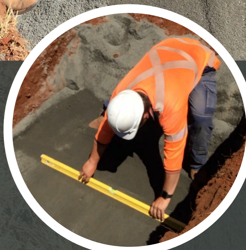
Ensure base material is compacted and level
