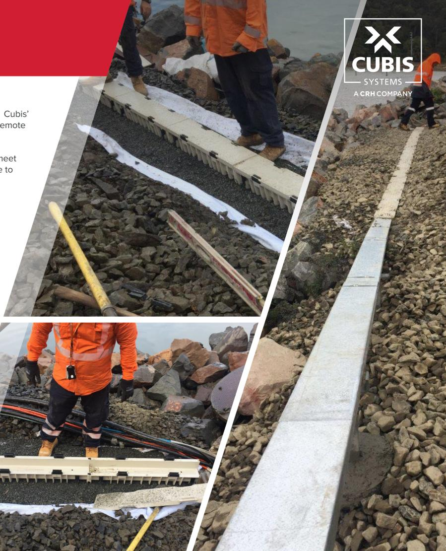
Superior asset protection was provided by the troughs interlocking tamper proof covers with secure locking bolts fitted on both sides. All remediation requirements, including excavation, assembly, integration with existing trough network, modification to the units and backfill were completed within hours using only standard power tools and no specialist labour or equipment.
